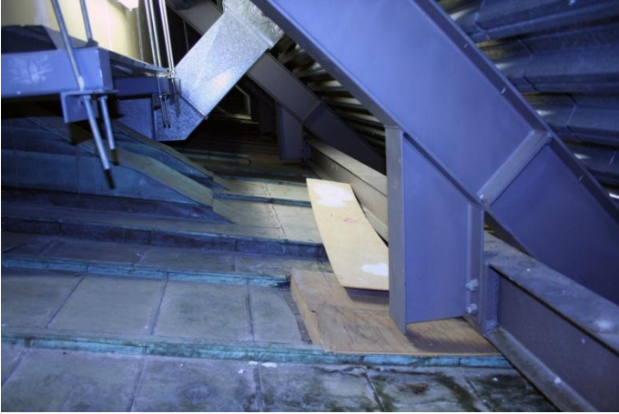
Original roof surface, and later 1993 roof structure
