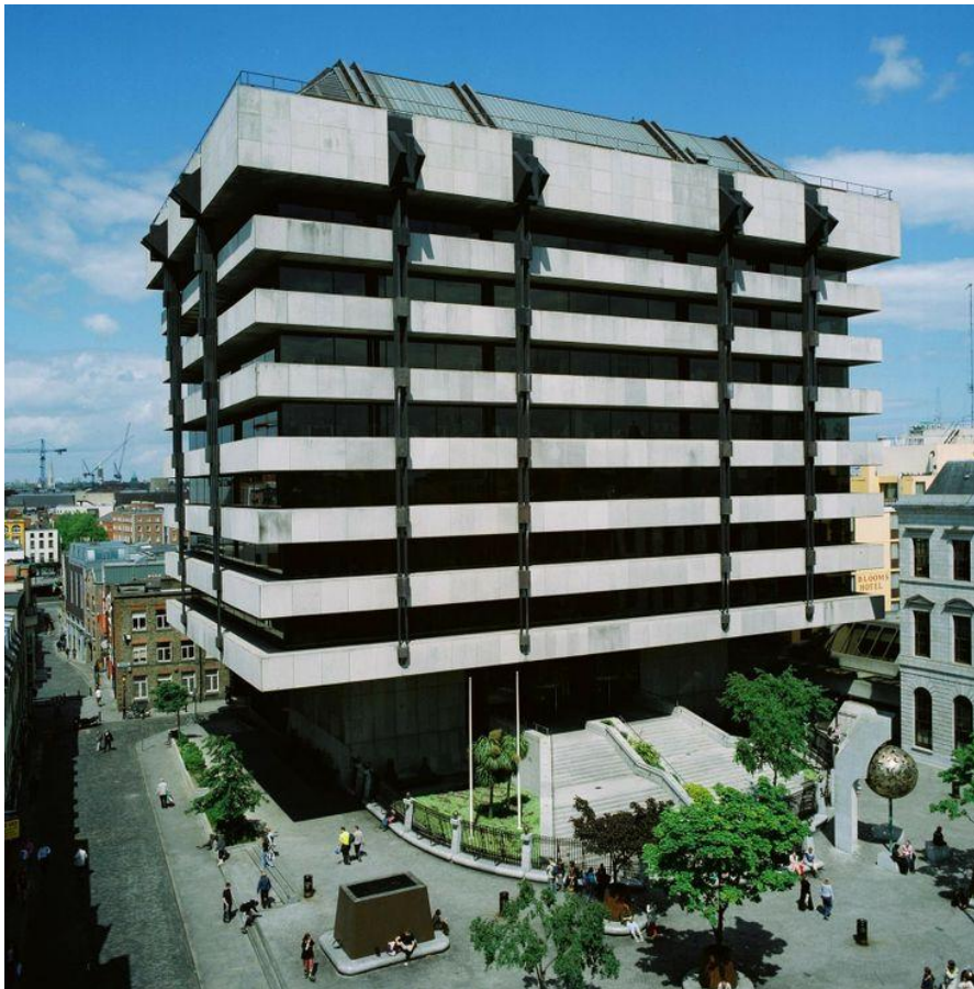
Photo of Structure
